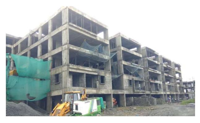
Block D1: Second floor Level slab  $1^{st}$  half concrete casting 100% completed. Shuttering works & Barbending works for  $2^{nd}$  half of Second floor level 70% completed.
