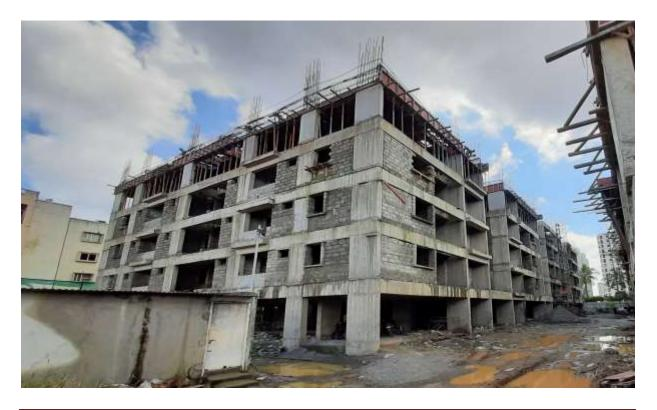
Community Hall: Shuttering & Bar bending works for Third floor level slab 65% completed and balance work on progress.
