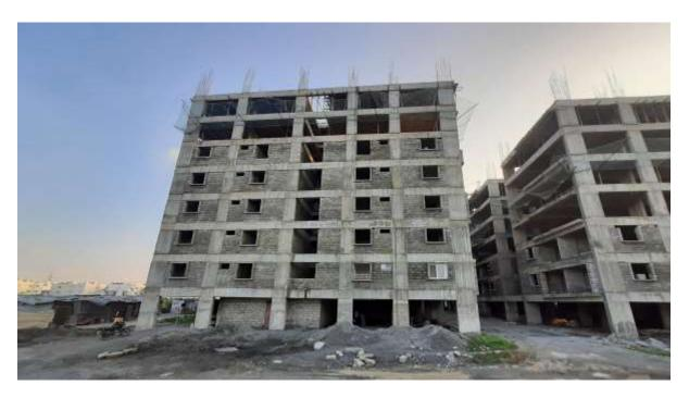
Block C2: Seventh Floor level slab First half concrete casting 100% completed. Shuttering and barbending works for 2<sup>nd</sup> half of Seventh Floor slab 70% completed and balance work on progress.
