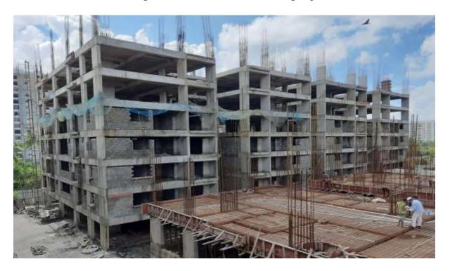
Block D3: Fifth floor level slab First half concrete casting 100% completed. Shuttering and barbending work for Second half of Fifth foor 40% completed.
