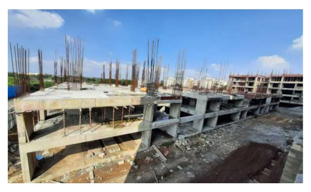
Block D2: Seventh floor level slab concrete casting 100% completed. Block work in Fourth floor 15% completed and balance work on progress.
