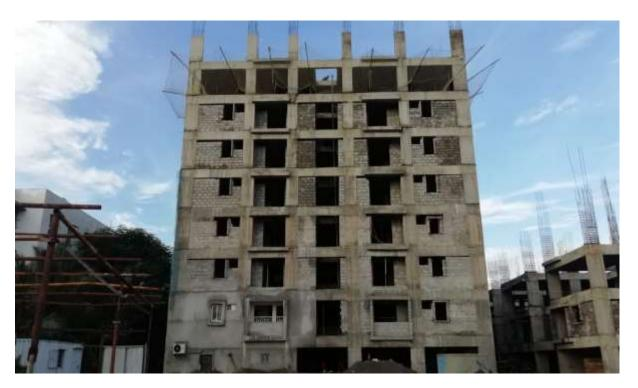
Block B2: Third Floor Level slab concrete casting 100% completed. Bar bending works for Columns up to fourth floor level on progress.
